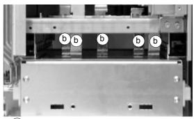
(b) M10x25 combi screws Tightening torque: 30...44 Nm (22...32 lbf ft)
